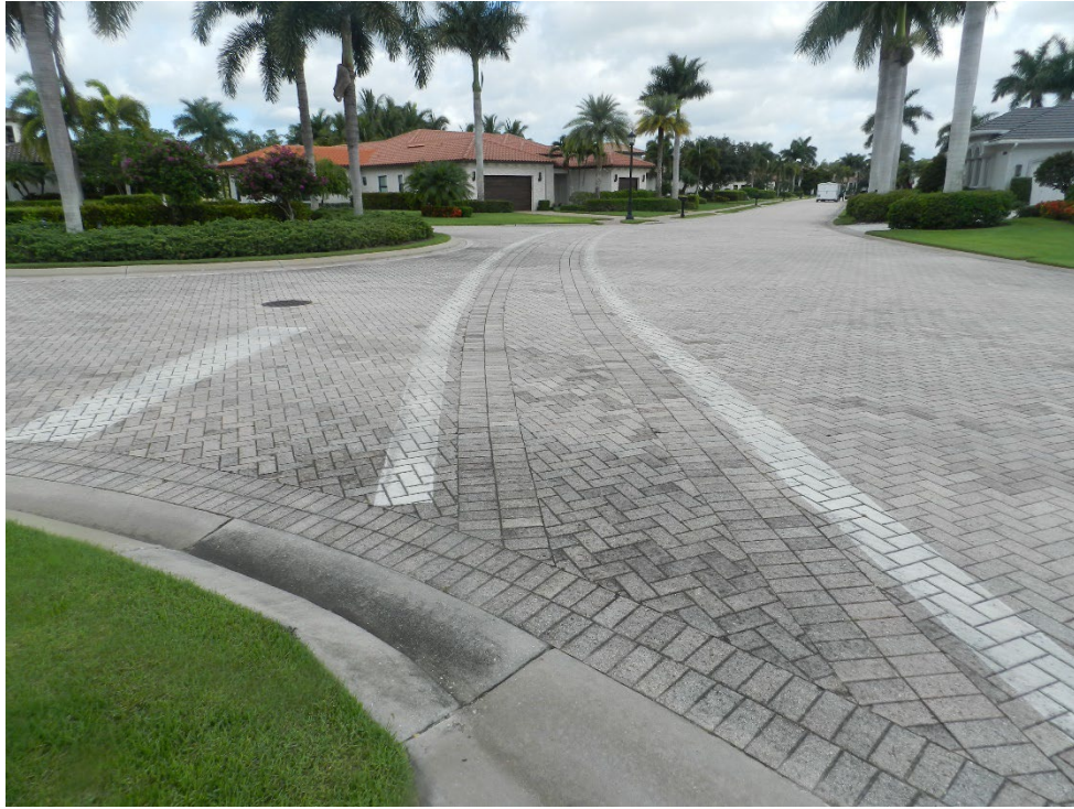
View of interlocking concrete paver roadways.
