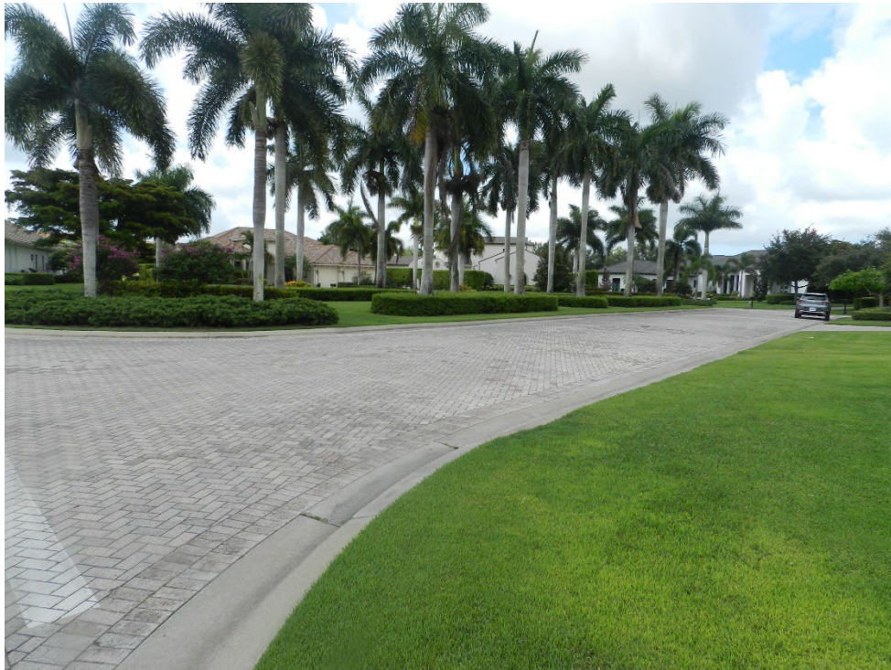
View of interlocking concrete paver roadway and typical common area landscaping.
