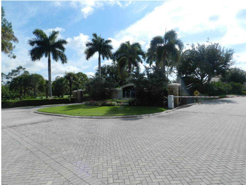
Entrance fountain structure, entry/exit gates, and interlocking concrete roadway pavers.
